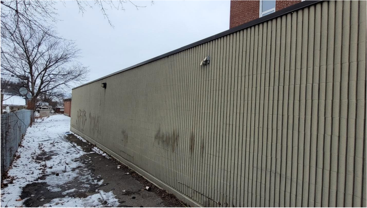
(Fig 5) (windows to be added to create residential studio apartments)(part of north elevation)
